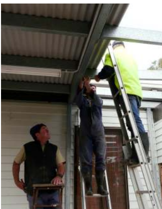
Working bee removing part of verandah
