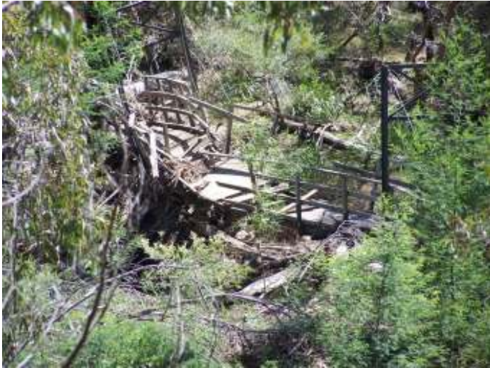
Walking bridge at Zumstein – ParksVic photo
